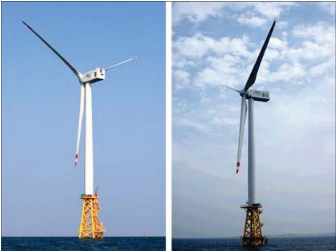
Figure 19. 3MW prototype wind power generator offshore Jeju Island, Korea
