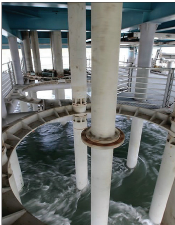
Figure 21. Tidal current power plant in Korea.
